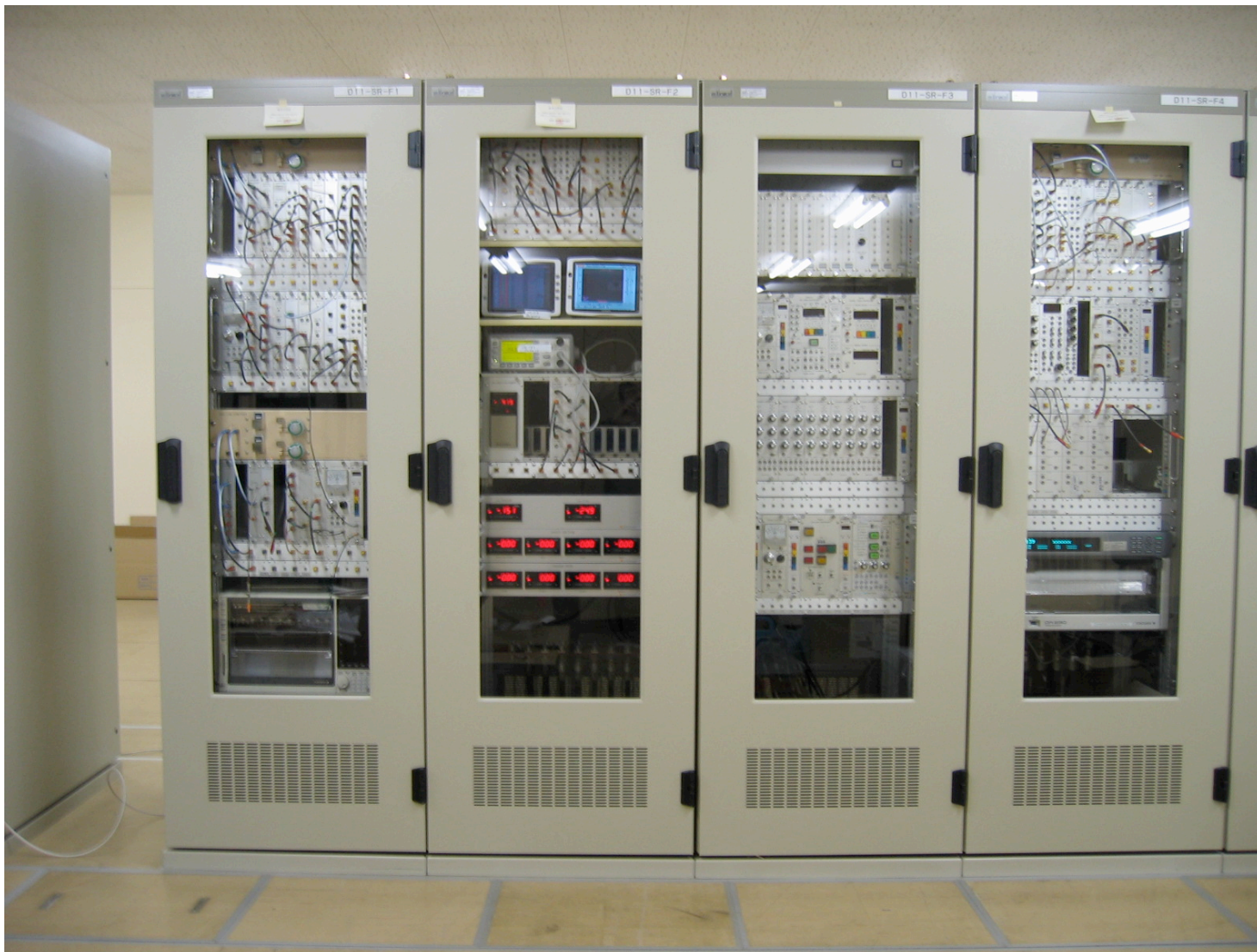
Commissioning of Crab RF system (K. Akai)
