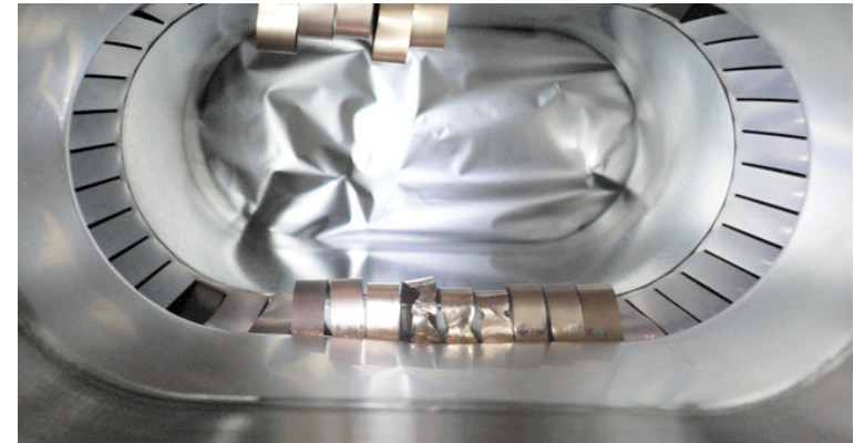
D03 broken bellows
