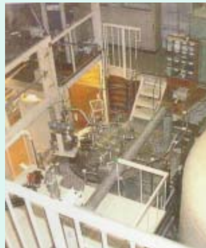
The crab cavity is set in the vertical cryostat
