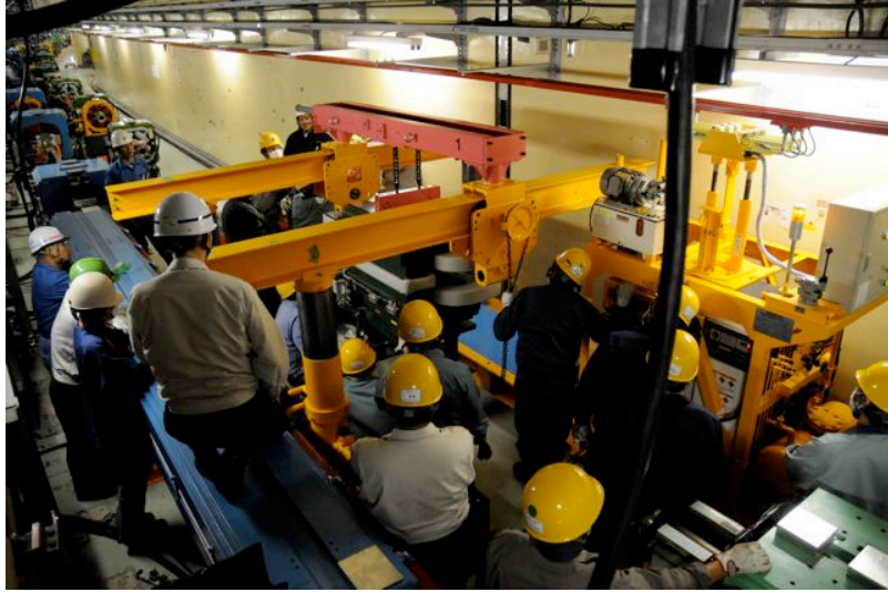
Removing LER bending magnets (107 magnets all done)
