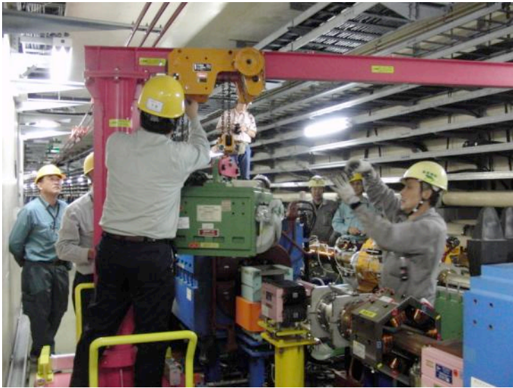
Removing LER beam pipes from Q magnets
