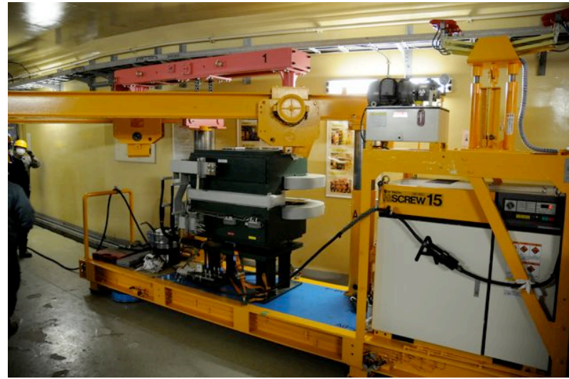
Removing LER bending magnets (107 magnets all done)
