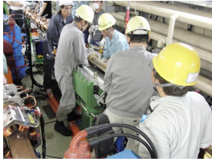
Removing LER beam pipes from Q magnets
