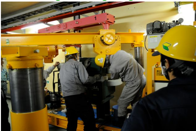
Removing bending magnet
