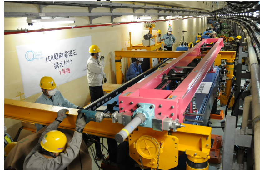
Install test in the outer LER over existing magnets in the inner HER.
