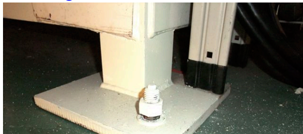
Anchor bolts at cooling tower released
