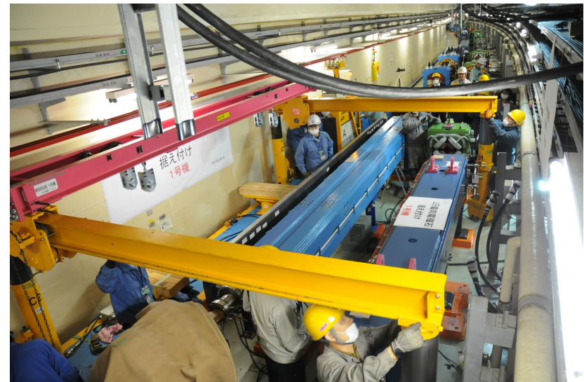
Install test in the outer LER over existing magnets in the inner HER.
