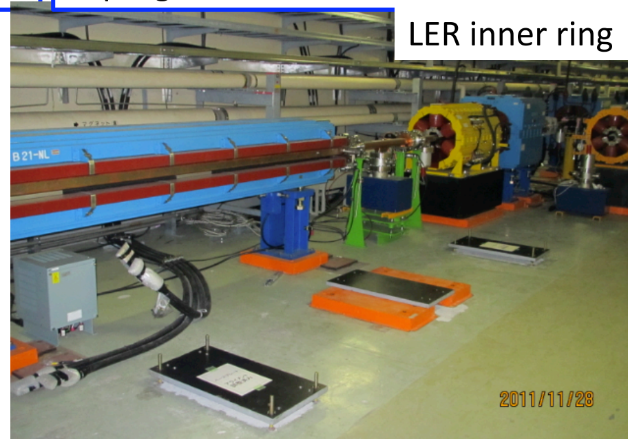
3.B) Base plates (3/dople) installation in progress.
