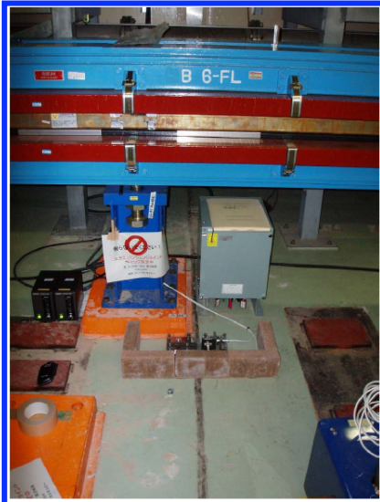
Monitor GAP distance at expansion joints
