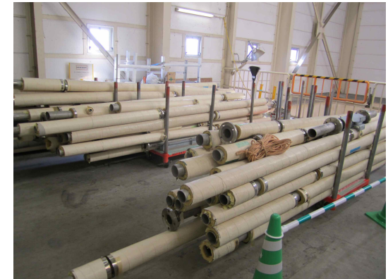
Cooling pipes removed from tunnel
