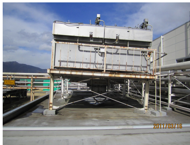
Air-fin cooler for klystrons
