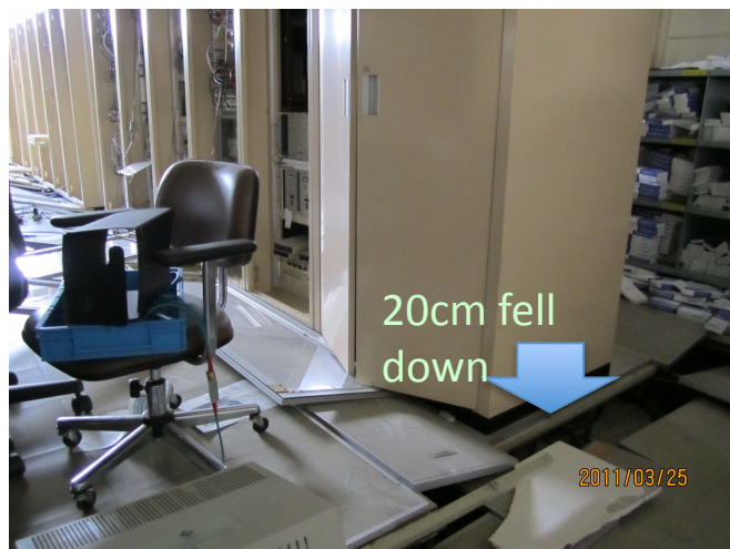
RF control system
