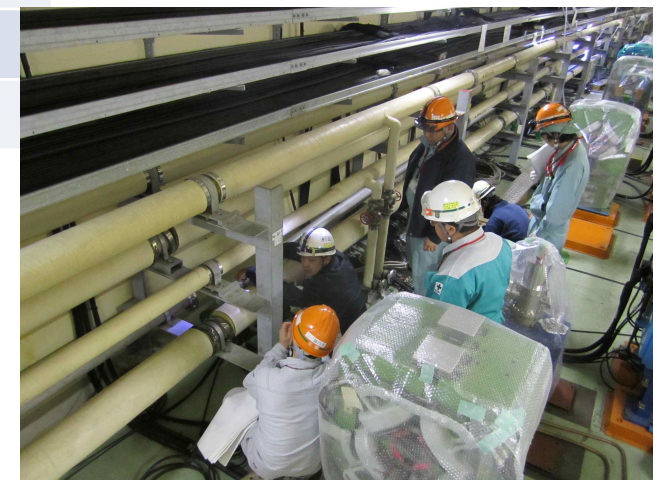
Replacing cooling pipes in the arc section
