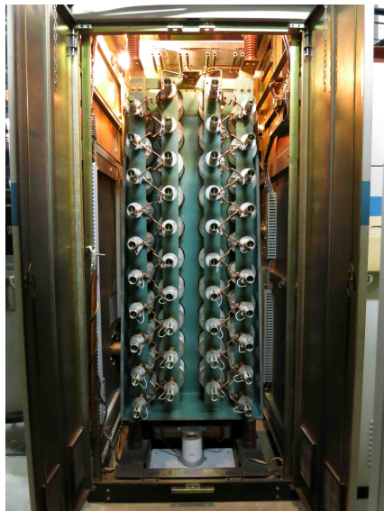
Klystron modulator PFN unit
