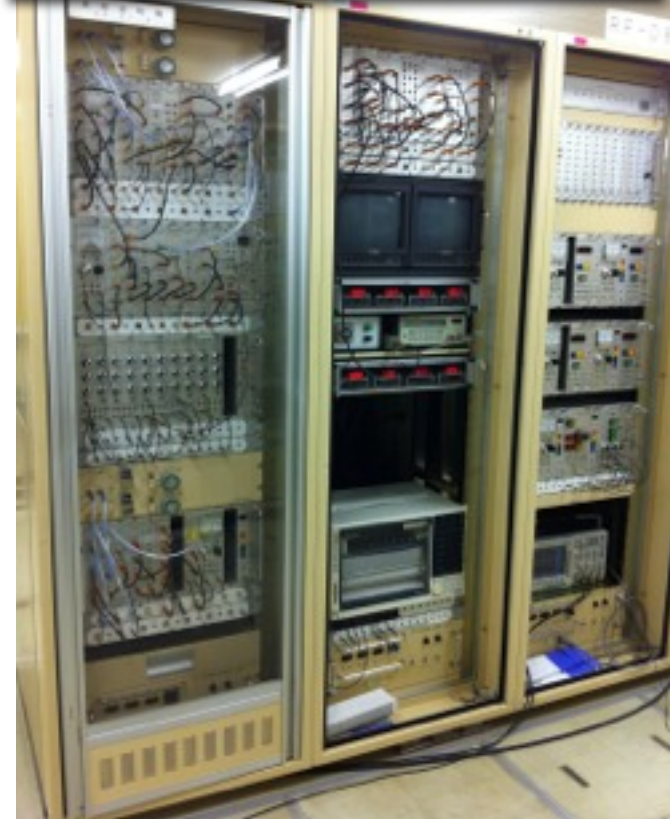
Present LLRF System of the KEKB ( for one klystron )
