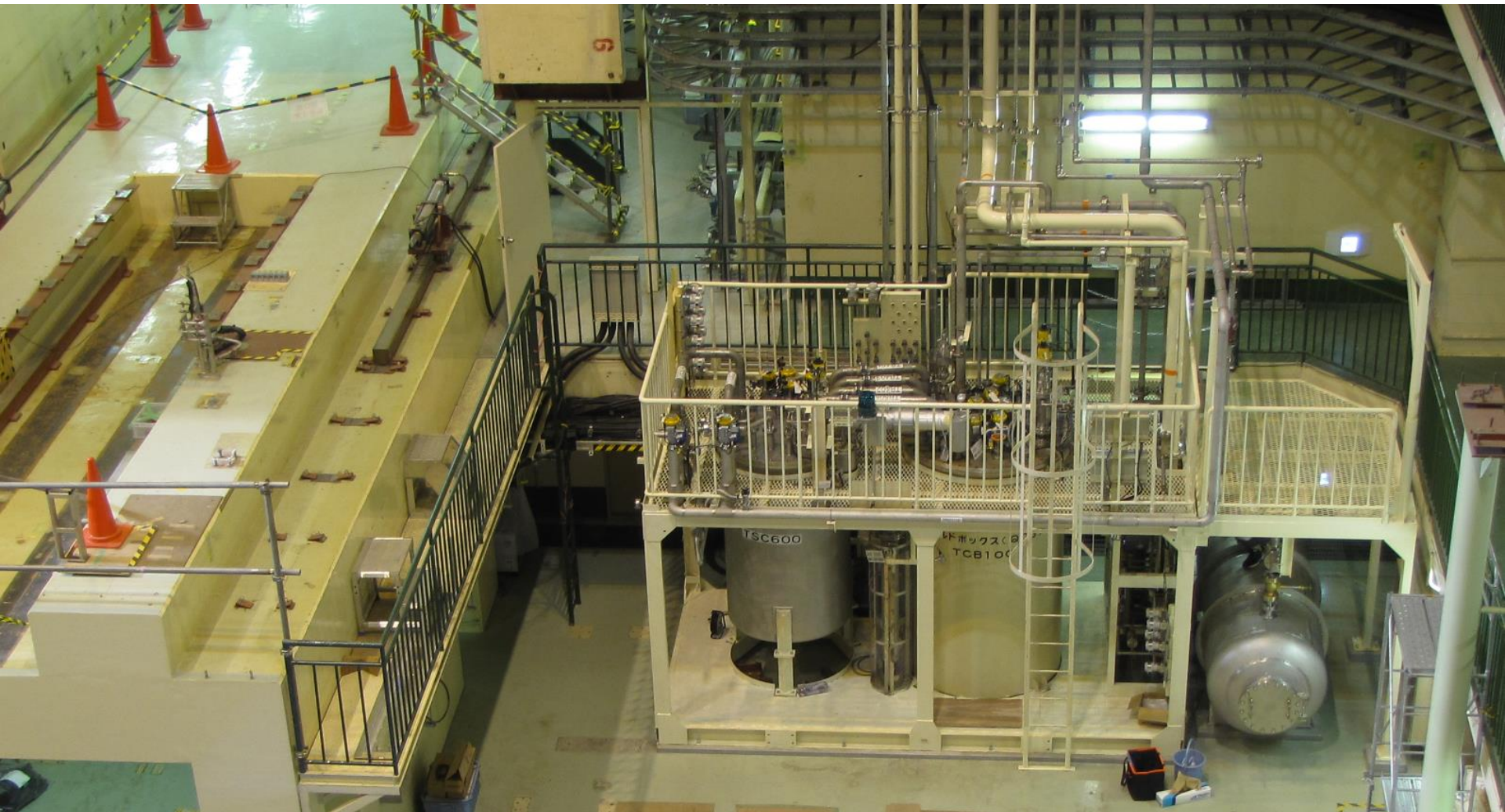
Cold box and subcooler unit
