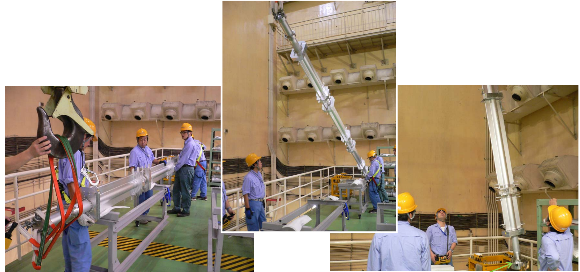
Hinge assembly to get beam pipe upright
