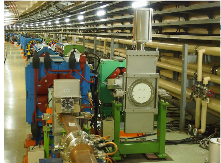
LER Gate valve in West tunnel
