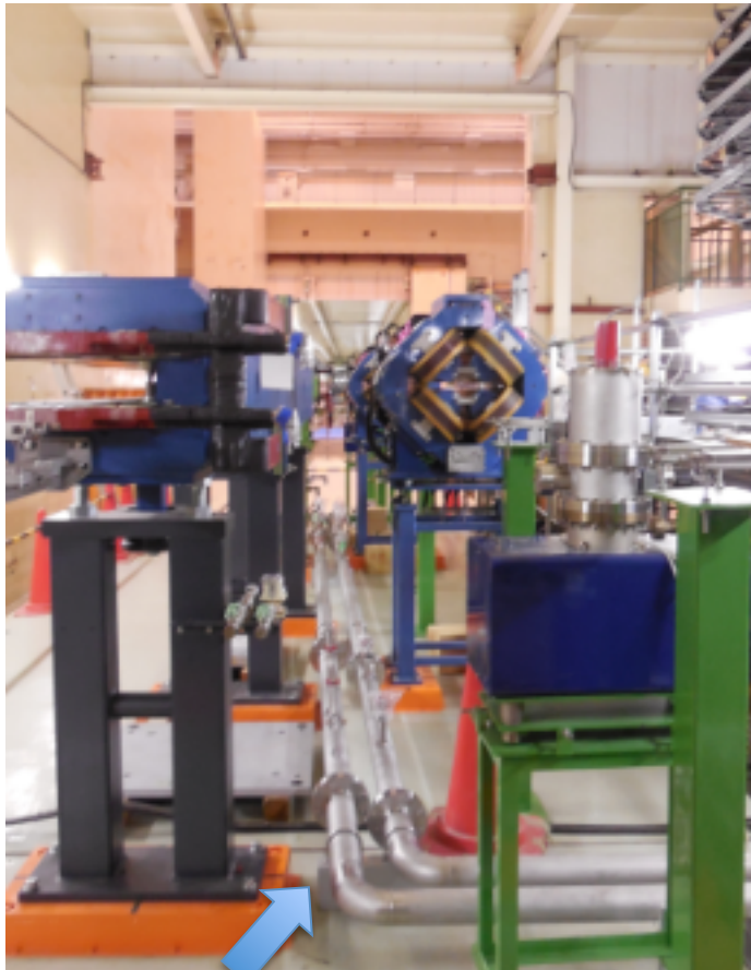
Part of the cooling water pipe lines being installed.
