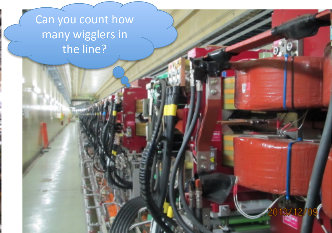
Power cables between wiggler magnets have been connected in the Oho and Nikko straight sections. Wiggler polarity has been checked.
