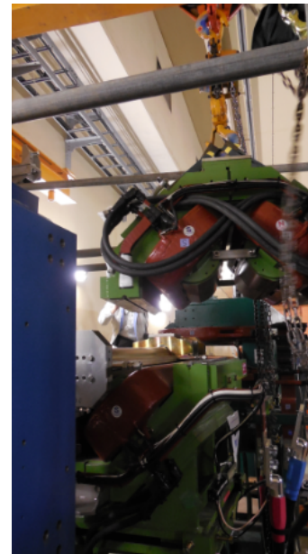
Removing the top half for vacuum pipe installation
