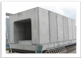
Gate shape concrete shields for the IR
