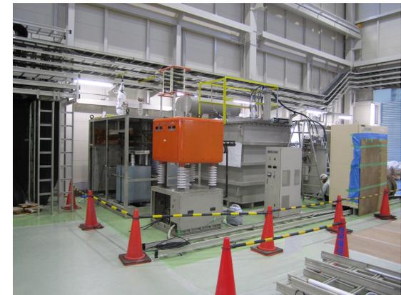
power supply for klystron
