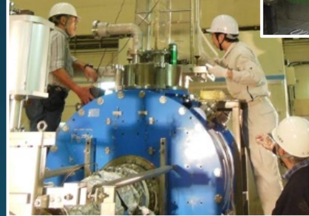
Before HHR, input coupler and HOM dampers were dismantled in a clean booth.
