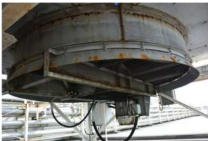
Corrosion of cooling fan for RF system
