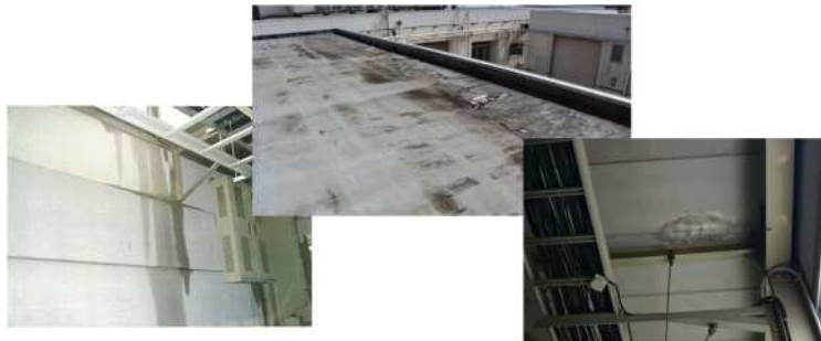
Water leak of MR power supply building
