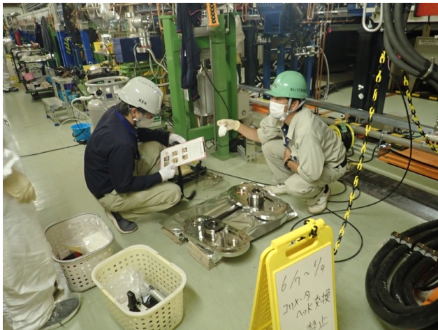
Clean the inside of the flange and chamber to remove deposits such as activated dust.
