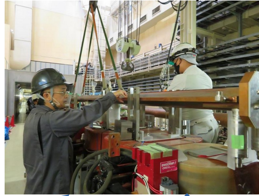
Remove vacuum pipes
