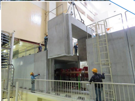
Concrete shield disassembly work
