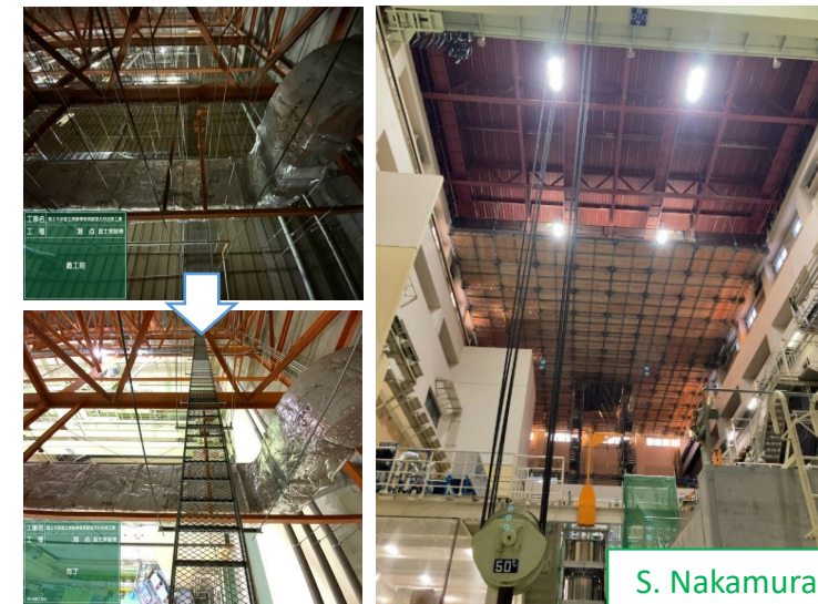
Ceiling aseismic reinforcing work
