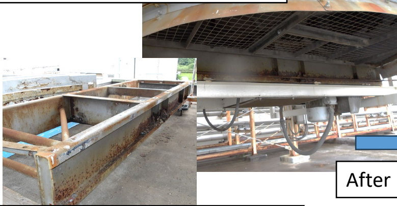
Beam for mounting cooling-fan
